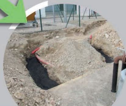
Anodes installation on coke breeze bed
