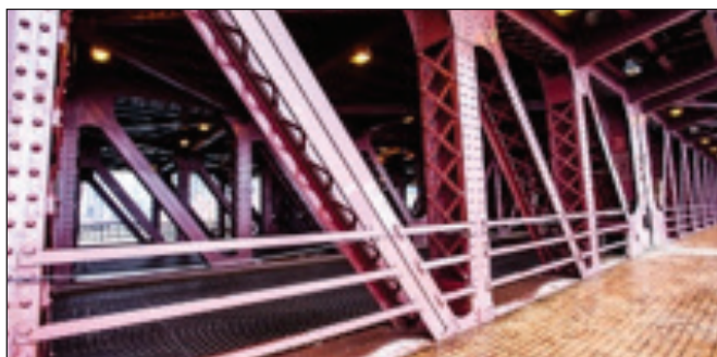
Person certification for steel engineering regarding corrosion control.
