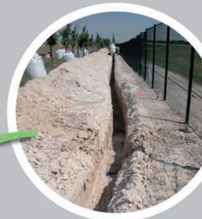
Anodes installation on coke breeze bed
